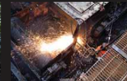
We Energies Coal Conveyors
